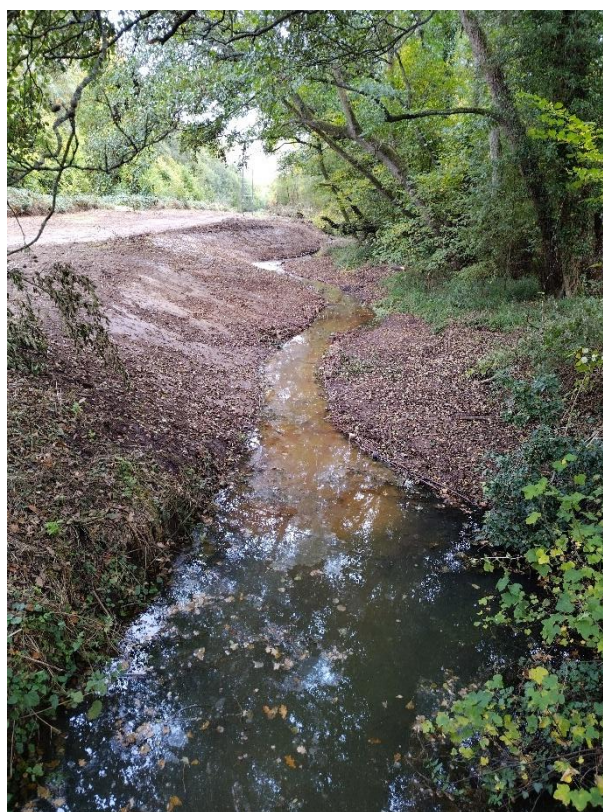
Reprofiling and opening up of the Sulham Brook at Moor Copse © Debbie Lewis
