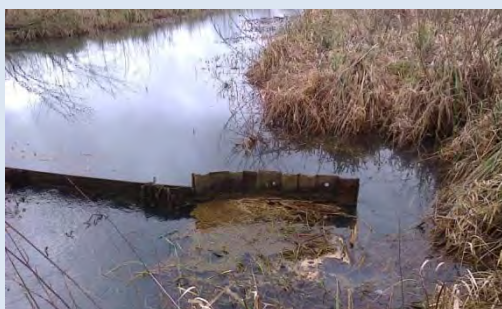
Fig 3a: Main weir on Middle Ditch, Feb'15, showing eroded by-pass channel (looking upstream)
