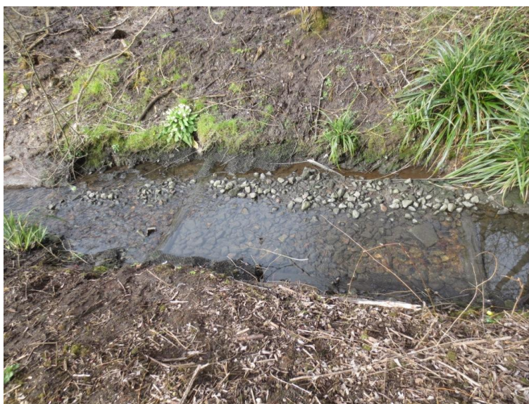
View of the limestone chippings and barriers installed in the brook bed to reduce bank erosion in 1985-88. Photograph 27.03.2015
