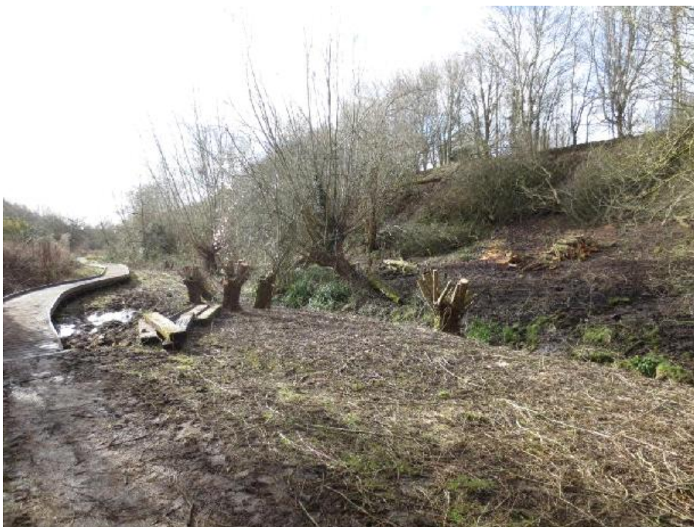
Re-pollarding of large outgrown willows and scrub clearance on the west side relic fen areas of LWS/LNR below bank to Warren Crescent. Note new plastic boardwalk now extends further to the north over cleared springs 29.01.2015
