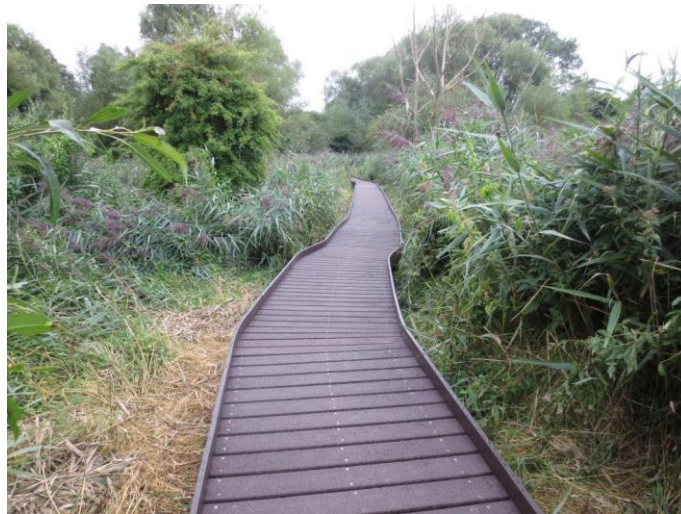
Before recent work, looking south, newly constructed boardwalk through still dense tall reed, 06.09.2013.
