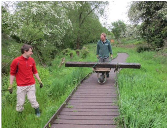
Wild Oxford work party. Moving old railway sleeper from original boardwalk down to pond area to use as bunding barrier to re-wet peat, 21.05.2016
