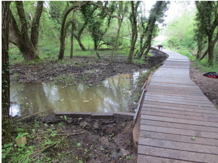
Board, railway sleeper and peat bunds on west margin of boardwalk retain iron oxide spring water previously lost. Dry peat area being re-wetted to the west and north. Removal of most of the willow trees to the left next winter will make the area even wetter and restore further fen areas. 21.05.2016
