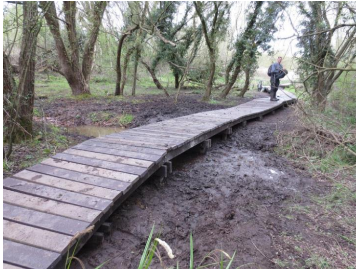
Boardwalk extension over the area of iron oxide spring flow that had previously required under-drainage to make the footpath passable (boardwalk extension on 01.05.2016 by Oxford Conservation Volunteers work party).
