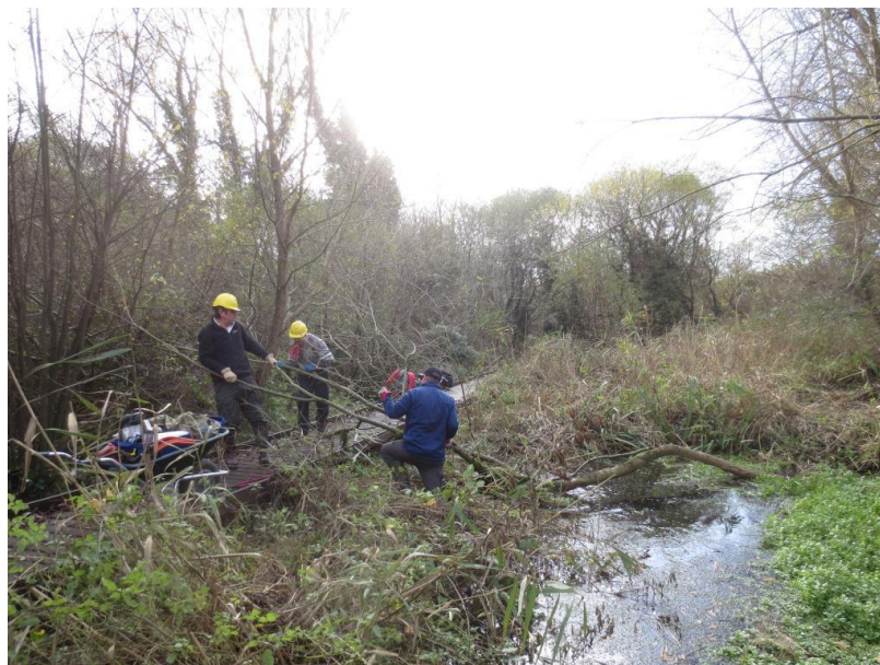
Cutting and removing shading crack willow scrub, 21.11.2015.
