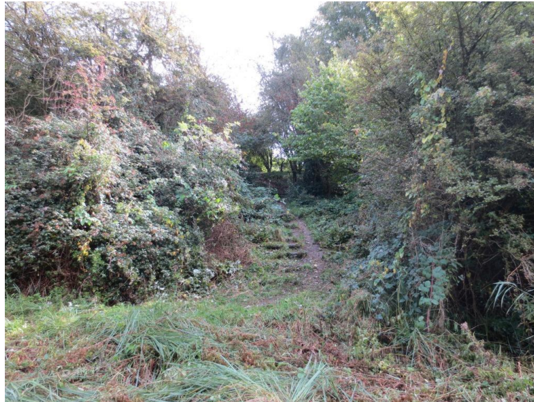
Before work, path steps were very steep and hemmed in by scrub 04.10.2012
