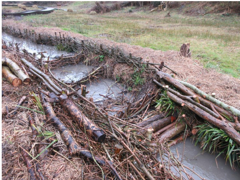
A sequence of a leaky log dam and several woven hazel wattle leaky dams, newly installed in the Lye Brook, slowing peak flow after rain on 28.03.2018. Bank erosion defence wattle structure with cut reed packed in behind is also visible.
