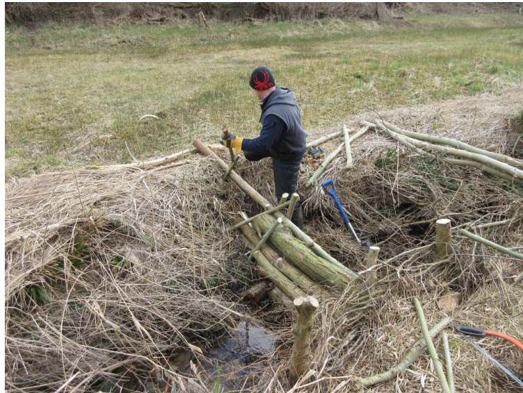
A leaky log dam in construction in the Lye Brook on 20.03.2018
