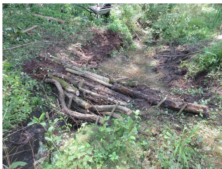
A log dam newly installed in the above area on 11.07.2019
